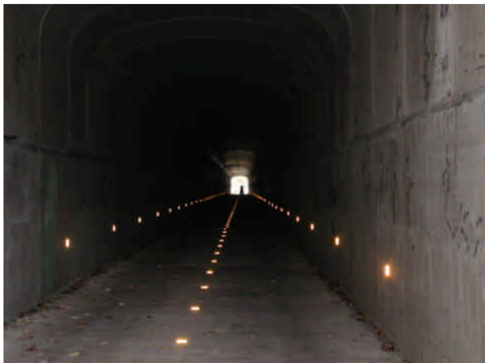
Tunnel on the bike trail
