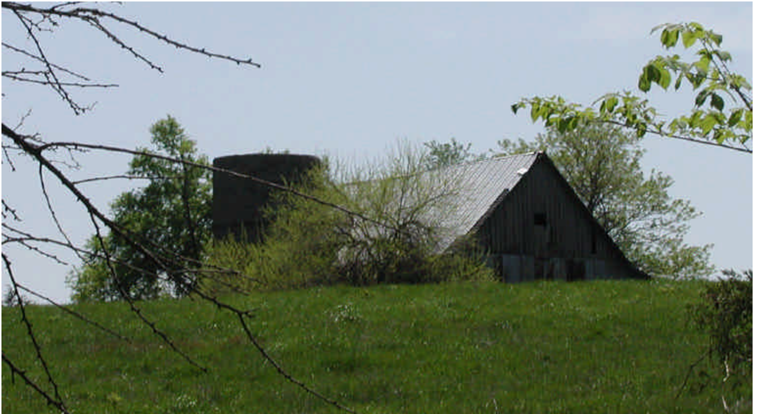
Cool old silos everywhere The Amish buy the old barns for the wood for their homes so you see the silos with no barns left These silos were built by pouring the first ring, raising up the form, pouring the second ring and up and up to the hight the farmer requested. They had an interior wood frame for the builder to work on and this was burnt before the roof was put on.
