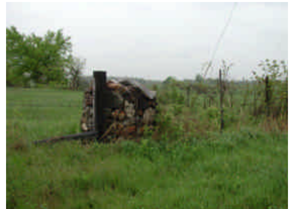
rocks are used for corner posts
